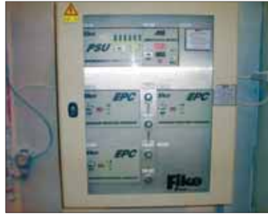
Part of Rebu's new ATEX-compliant explosion-protection system
