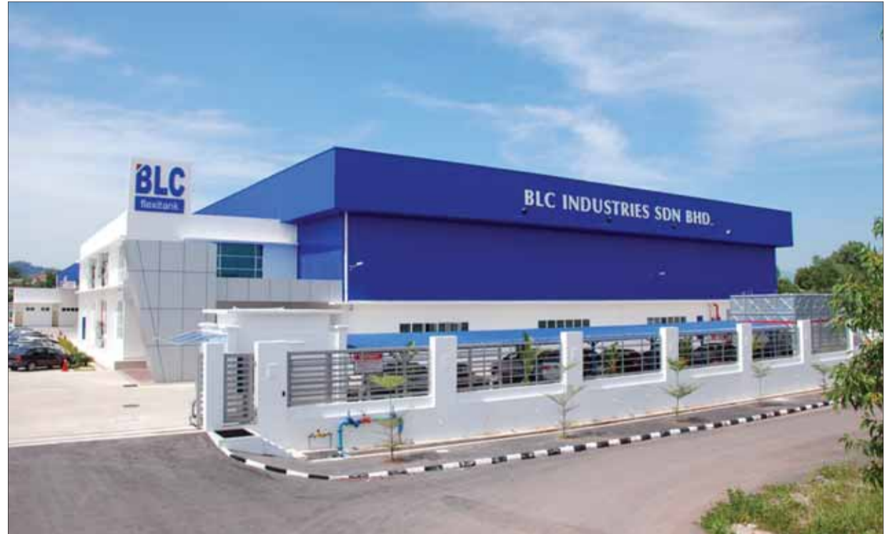
BLC's new facility: "conceived, planned, designed and constructed specifically for flexitank manufacturing"
