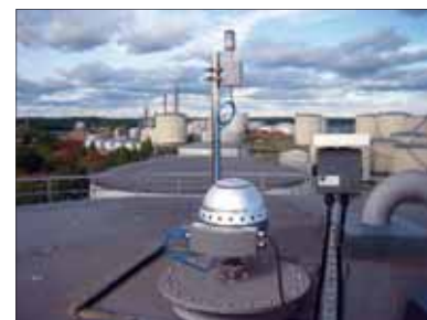
Rosemount Rex radar level gauges, equipped with Smart Wireless THUM adapters have been installed to replace existing mechanical servo gauges
