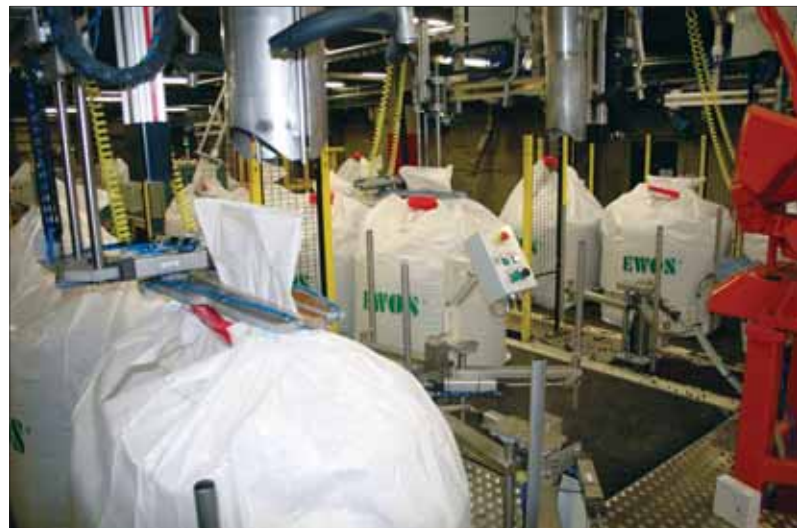
Three automated PORTABULK filling lines for fish feed installed at an Ewos plant in Norway
