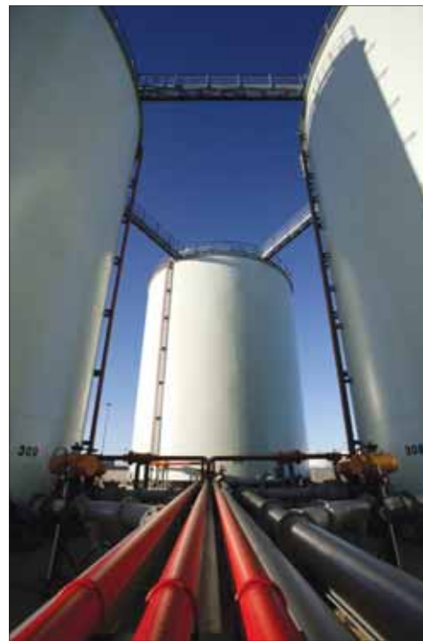
The Simon terminal has dedicated three tanks with a combined capacity of 4,000 cbm to the contract
