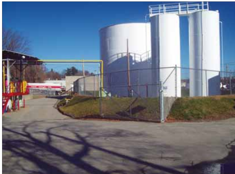
Dead River Company recently upgraded the automatic tank monitoring and gauging systems on its storage tanks at three of its bulk plants to the SiteSentinel iSite Automatic Tank-Gauging System from OPW Fuel Management Systems
