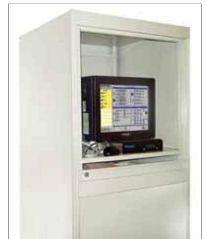
The OPW SiteSentinel iSite console and Petro Vend FSC3000 site controller located in one of Dead River's bulk plant facilities
