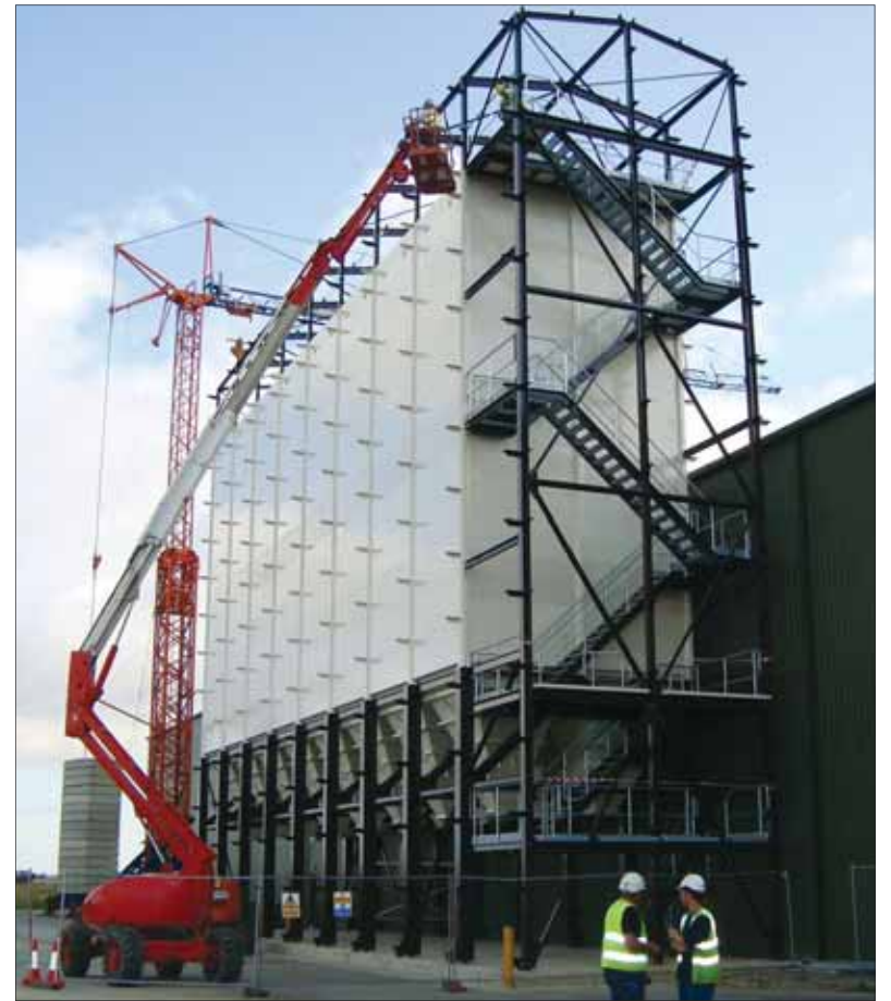
Working with GAME Engineering, SCE in 2009 installed this silo system for Waggs Foods in the UK
