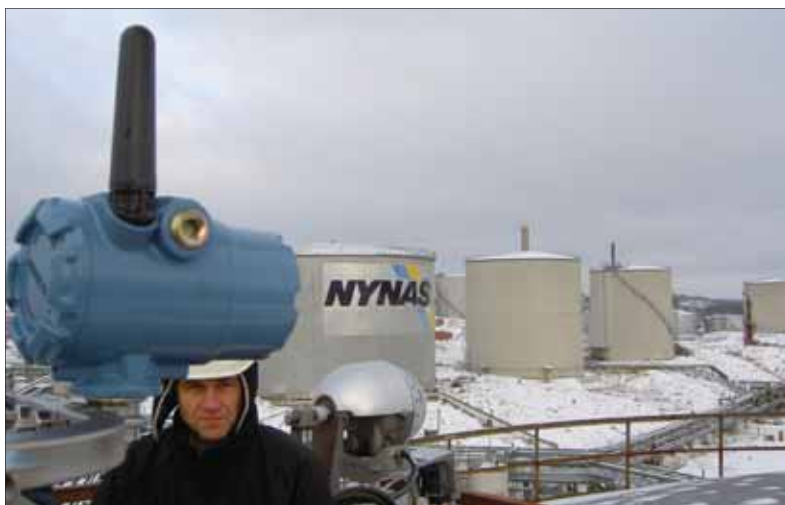
Rosemount wireless transmitters installed on large vessels act as repeaters
