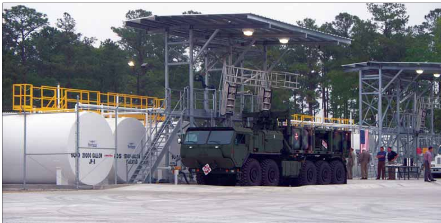
The racks were customised to accommodate vehicles varying in height as well as to withstand specific environmental conditions
