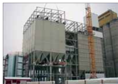
SCE's Wozniak silo installation approaching completion
