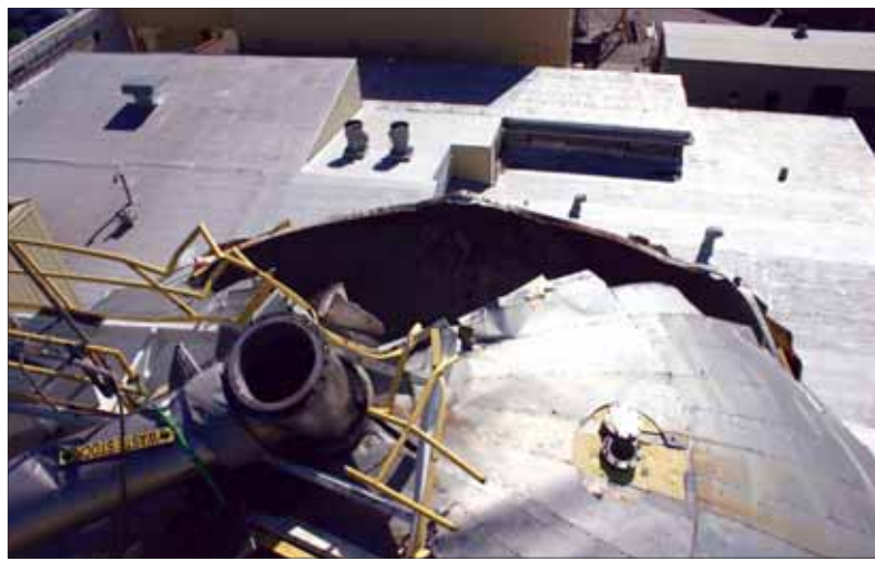
The CSB determined the explosion resulted from welding above an 80 ft tall storage tank that contained highly flammable hydrogen gas
