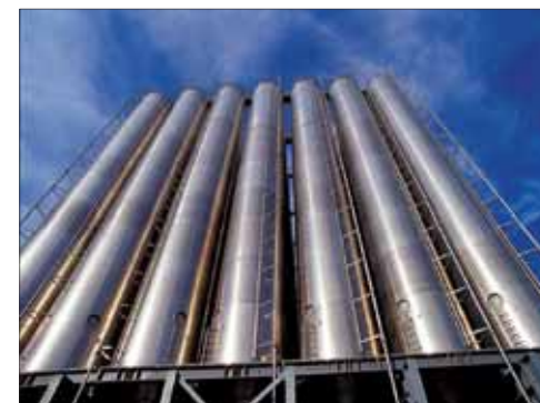
One of Greiwing's dry bulk silo batteries
