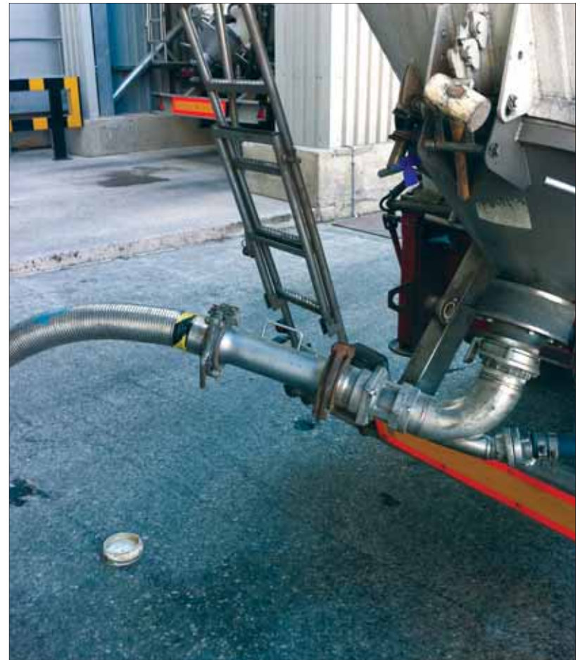
Greenwood Magnetics Anker Magnet fitted to a tanker line blowing our
