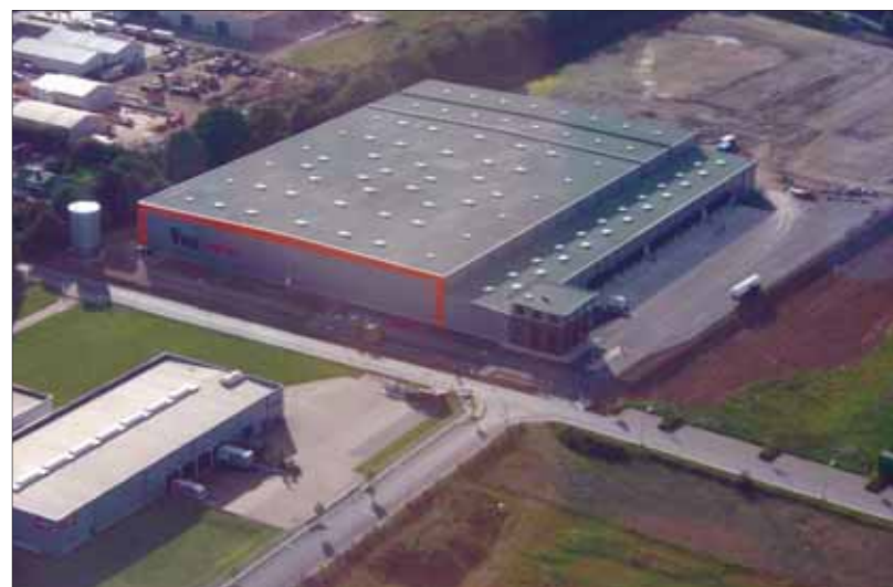
The Vos Logistics distribution centre in Goch, Germany is undergoing expansion.
