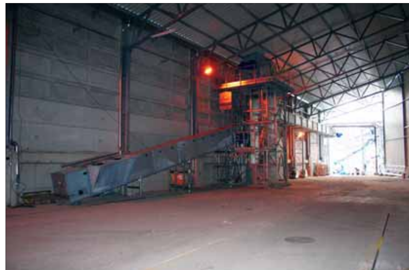
Cimbría Bulk Equipment has supplied a package of chain conveyors such as the one pictured belt conveyors and bucket elevators to Bunge's Swinoujscie grain transshipment facility
