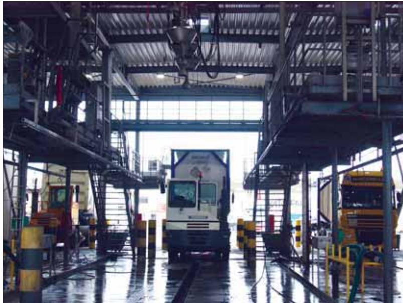
It not only takes care of the company's own waste water but also handles waste from other sectors
