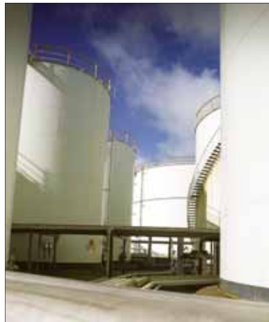
The contract at Simon's Seal Sands Terminal extends Harvest Energy's expanding UK-based storage and supply network
