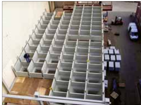
72 smooth-wall cells being installed by SCE engineers at ATR's new bulk distribution station
