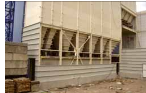
Extra SCE silo storage cells have been added to the Ostend production plant of Fides Petfood
