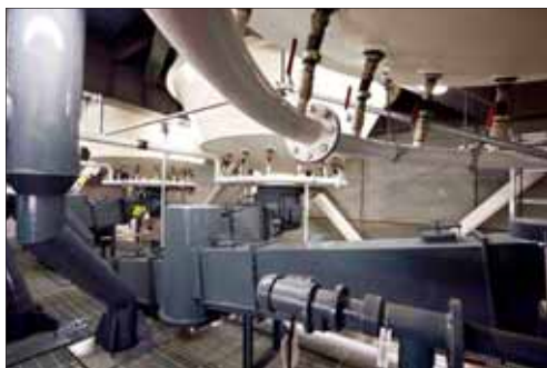
Silo discharge for truck loading, allowing a 30t capacity road tanker to be filled within 10 minutes
