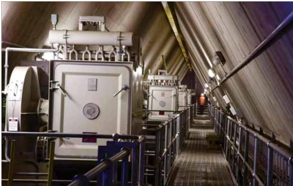
A reclaim tunnel extends along the entire length of the storage facility
