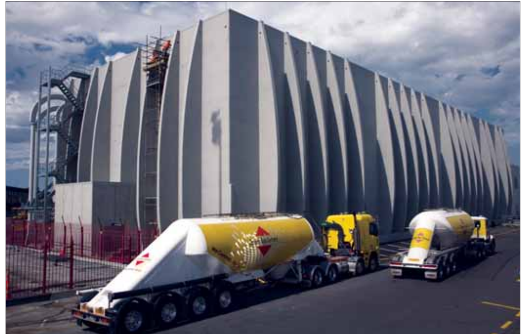
Golden Bay Cement's architecturally elegant Eastport cement terminal merges well with other buildings on the Auckland waterfront
