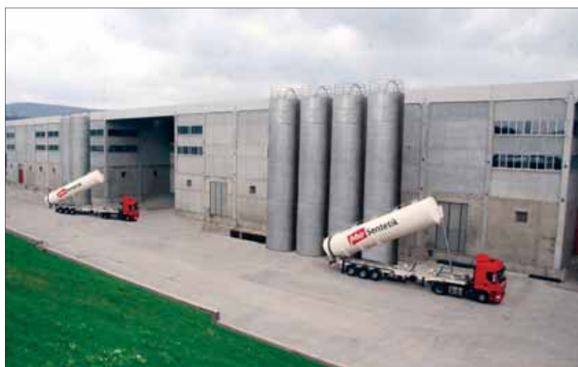
In order to keep stringent quality control of pharma FIBCs manufactured under sterile conditions, Isbir operates its own fleet of regularly cleaned road powder tankers which deliver polymer raw materials to the factory
