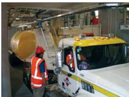
A cement truck in the process of being loaded: the fully automated loading sequence is managed by a SCADA computer control system
