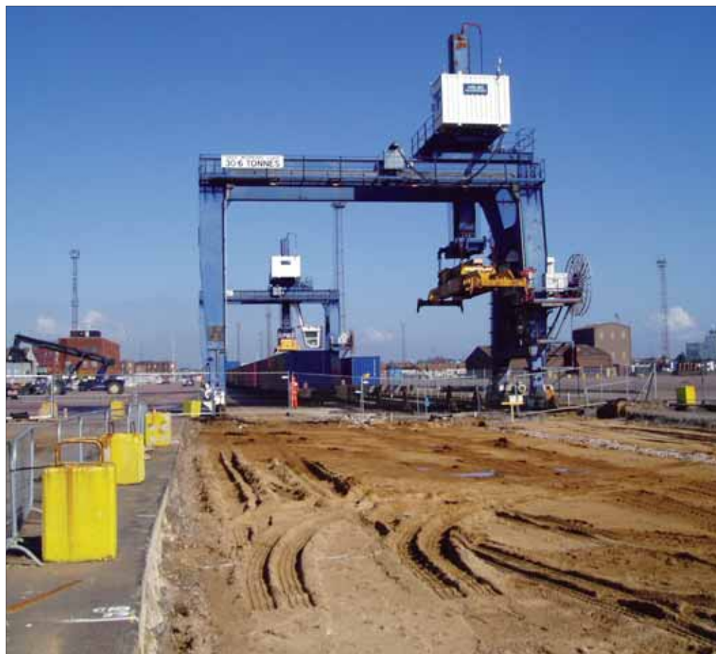
The South Rail Terminal was extended by 39m on all three lines earlier in the year
