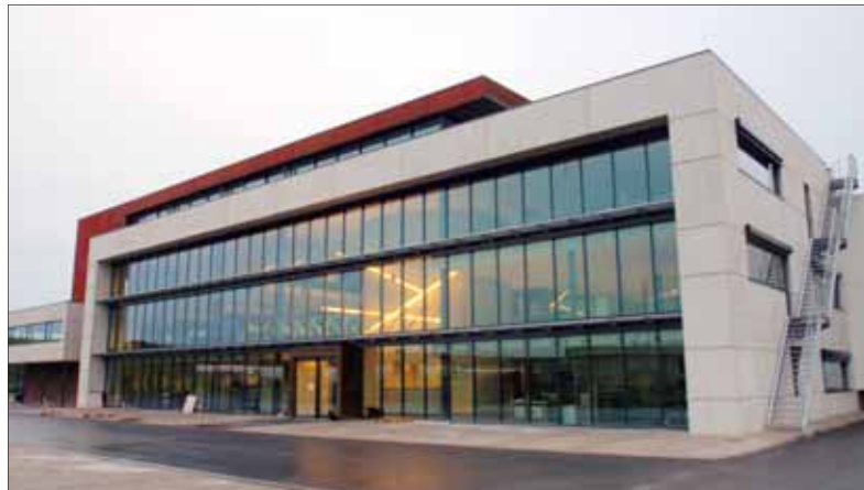
The new Ivens head office - exterior and interior
