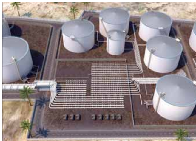
The terminal consists of 641,000 cbm of storage across 20 tanks
