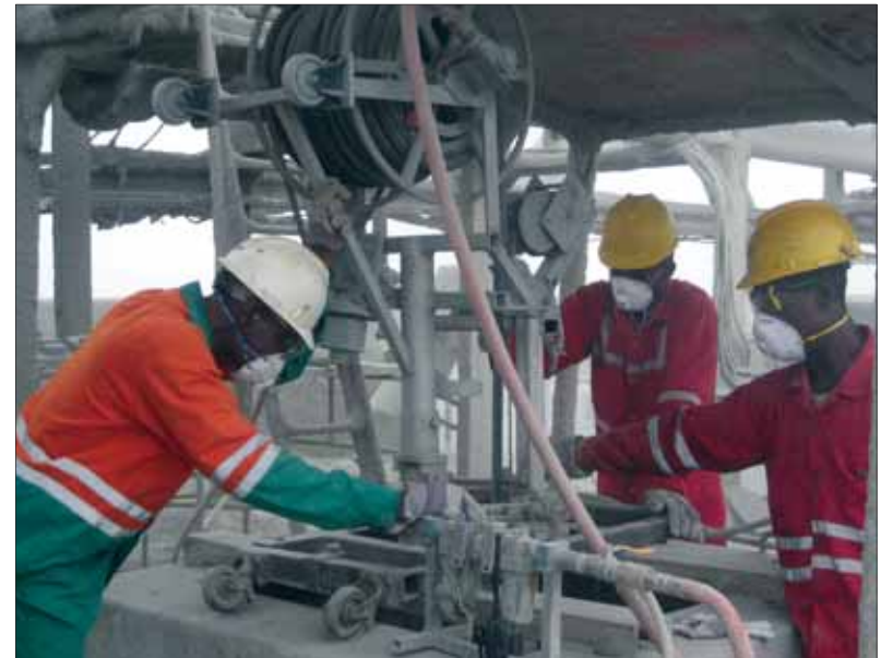
A Primasonics Prima Whip being operated at Lafarge's Sagamu plant
