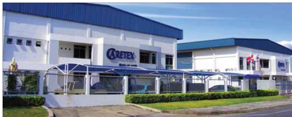
The Caretex liner manufacturing facility in Thailand
