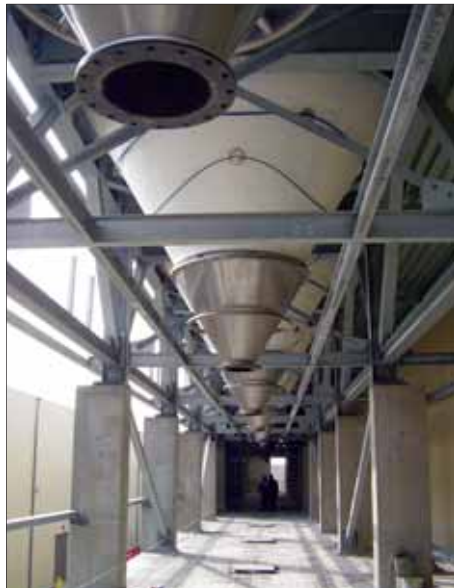
The Katoen Natie silo battery in Antwerp and (right) view of the discharge cones
