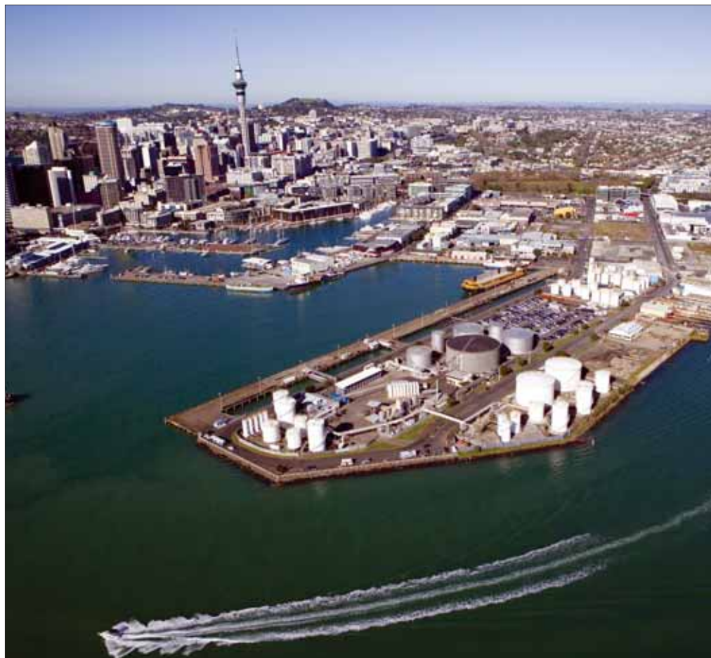
Marstel's assets include tanks in the Wynyard Precinct, Auckland
