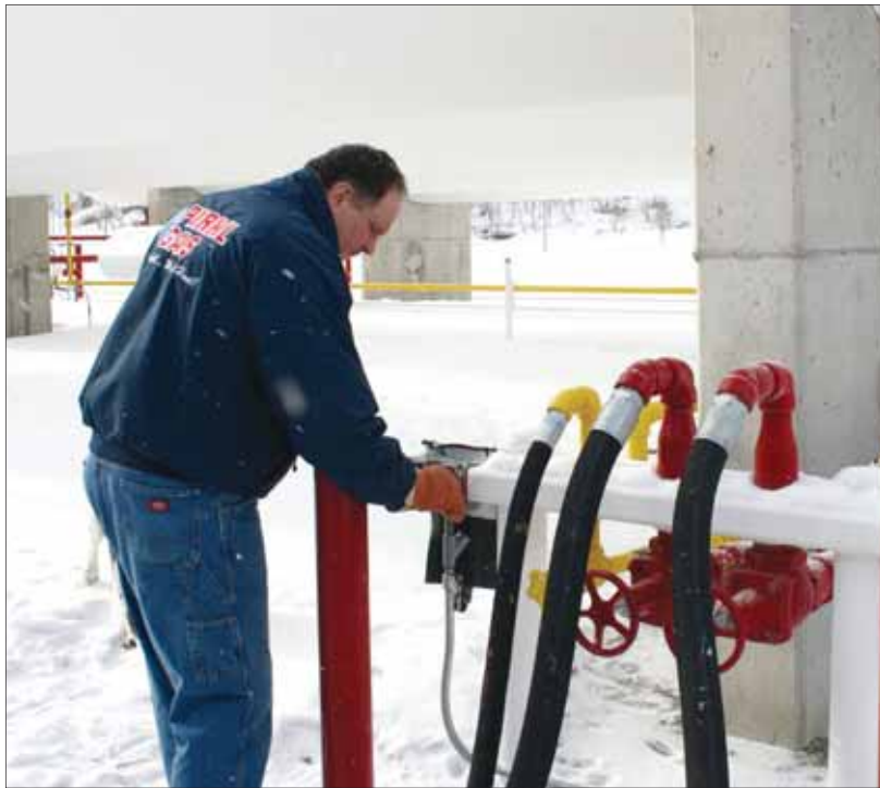
Greg Pirkl activates the shutoff valves at the recently upgraded bulk plant
