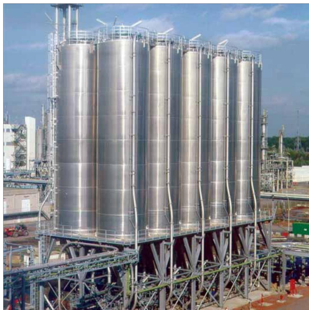
Typical Ellimetal aluminium silo battery of the type favoured by dry bulk logistics operators, providing third-party strategic storage and local distribution of polymers and chemicals for their customers
