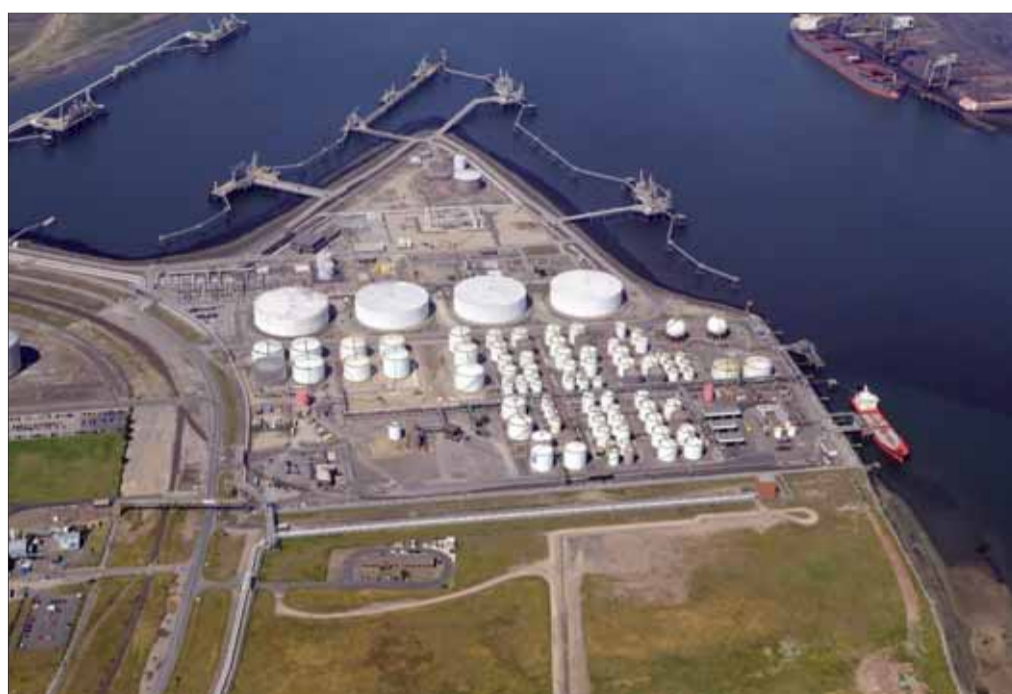
Simon's team was able to modify 10 existing tanks to the required specification in just 60 days
