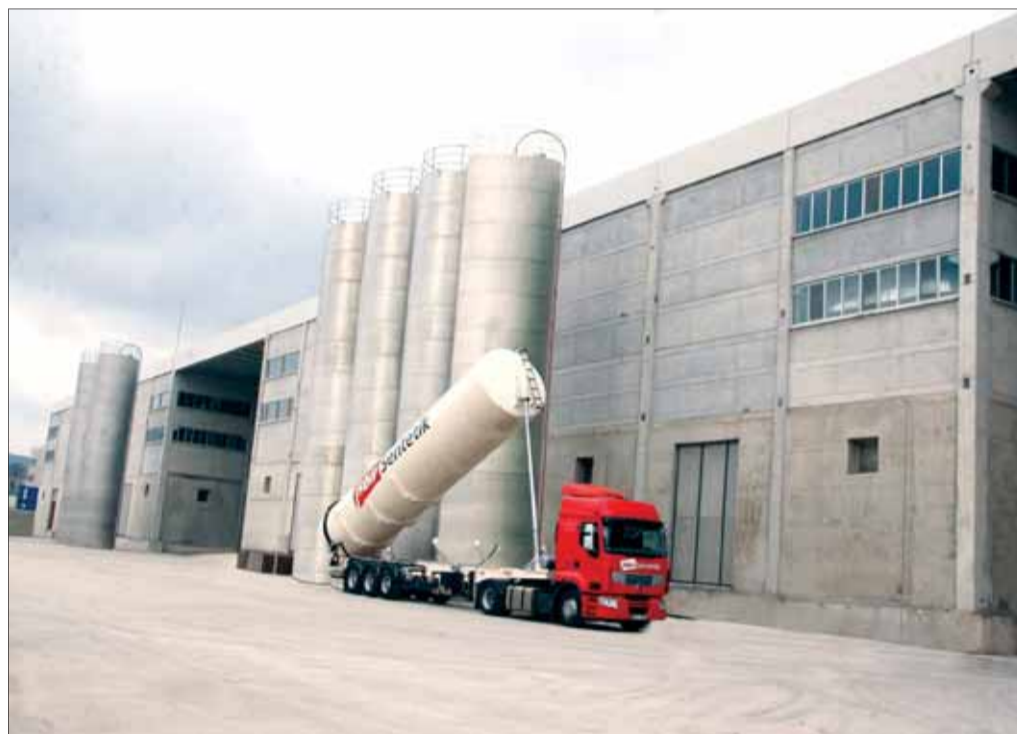
Stainless steel silos at the new Turkish bulk bag plant of Isbir Sentetik provide clinically clean storage of raw materials employed in clean-room manufacture of the bags; the materials are delivered to the plant in special road tankers internally lined with stainless steel, allowing the powders/granulates to be maintained under aseptic conditions at all times
