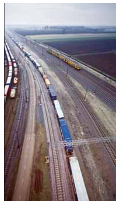
Full liberalisation is critical to the success of rail freight
