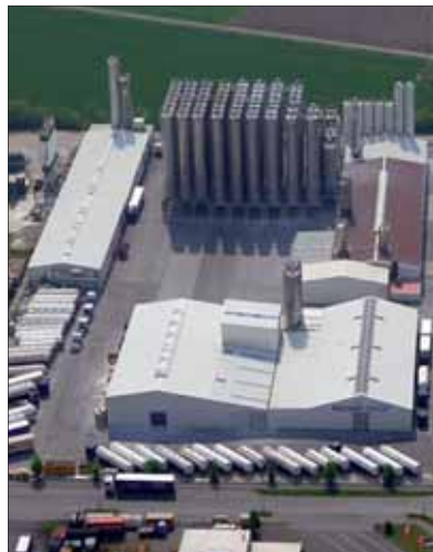
Aerial view of Greiwing's new granulate pilot plant, showing the two main buildings and the silo battery
