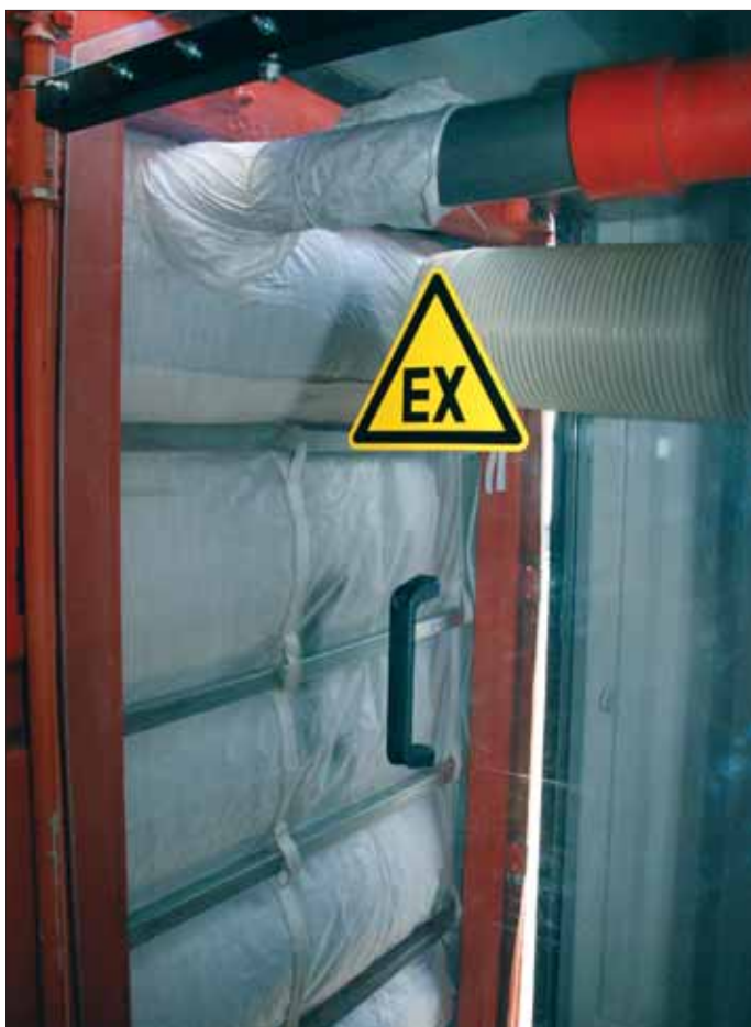
The filling pipe protrudes into the specially designed liner to ensure virtually contamination-free transfer of the bulk cargo
