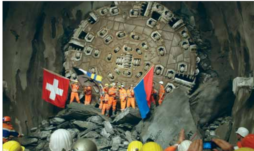
The drilling may be finished but there's still a lot to do
