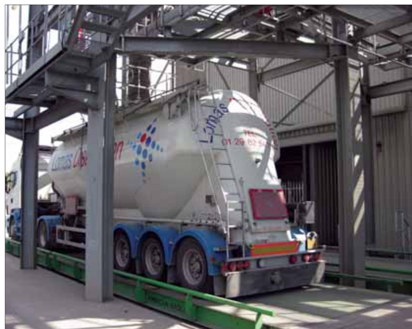
The Precia-Molen automated loading and weighing system at RockTron's new Fiddler's Ferry eco-mineral processing plant
