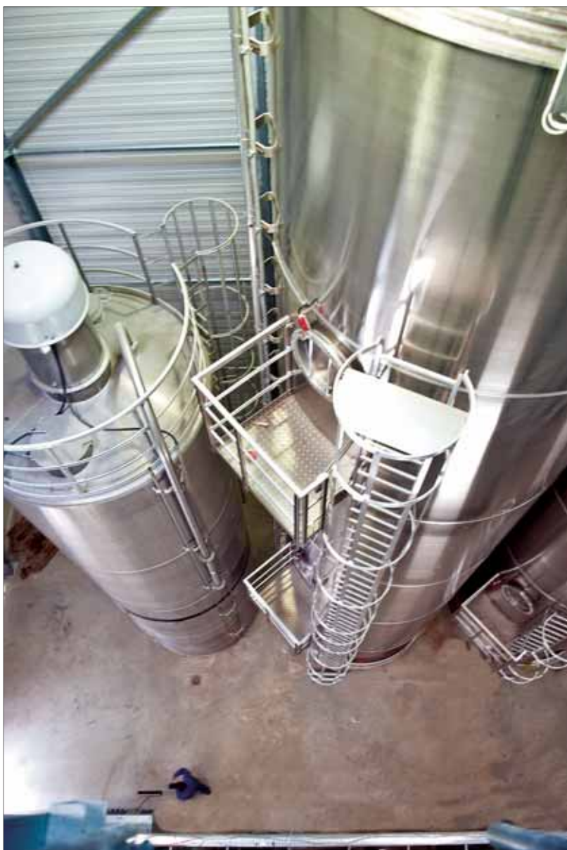
Apart from the main silo battery, there are various individual storage silos some of which are exclusively available to customers on a hire basis; the vessel shown on the left is for individual small batches
