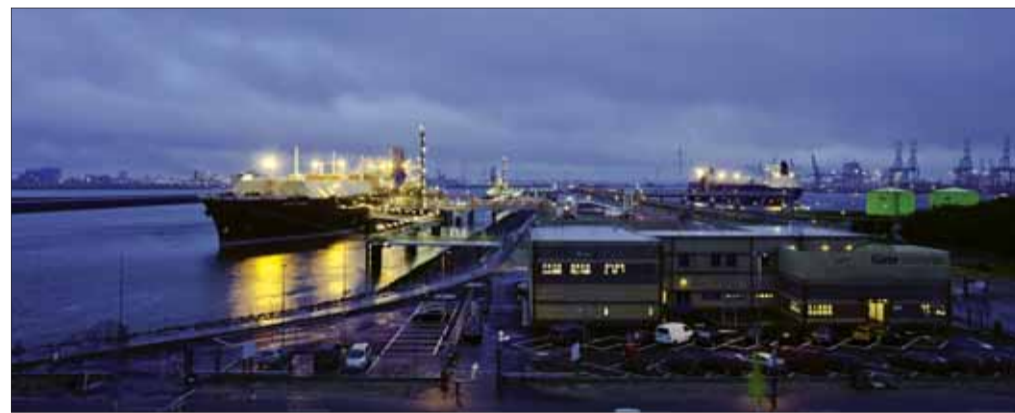
Throughput capacity of Gate Terminal is 12 billion cbm a year
