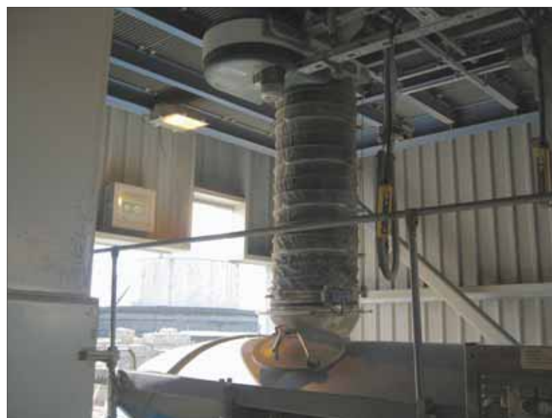
Cimbría Moduflex chute loading cement into a road powder tanker
