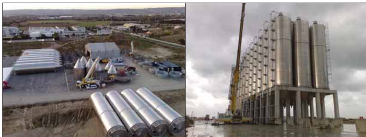
Employing its new silo assembly system, Ellimetal completed this project well ahead of schedule despite bad weather
