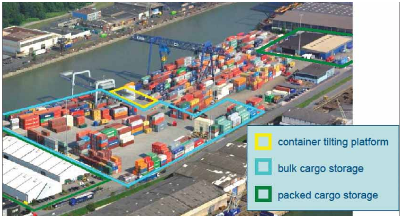
Aerial view of the new Schmidt/Imperial plastics distribution facility at the Rhein-Ruhr Terminal showing bulk container storage, warehousing for bagged products and the location of a new container tipping platform
