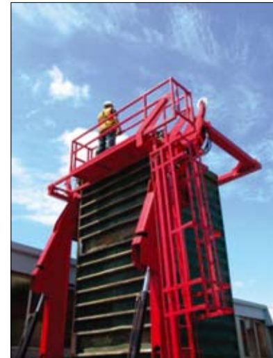
Once the container is tipped the worker has easy accessibility to the top
