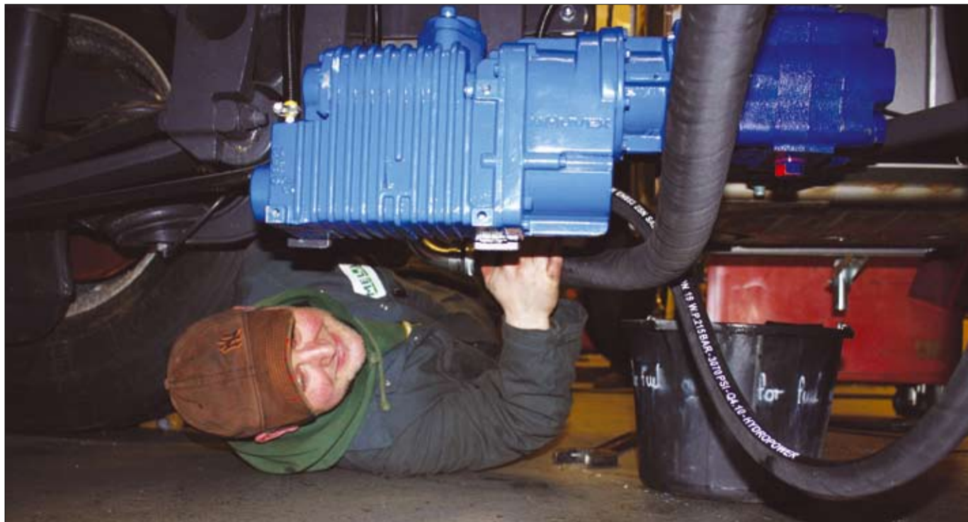
Meller Flow Trans (MFT) installers prefer the lightweight, compact size of the B200.
