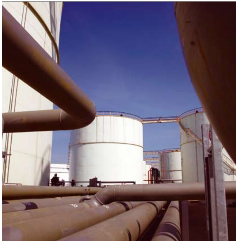
Simon Storage Seal Sands terminal
