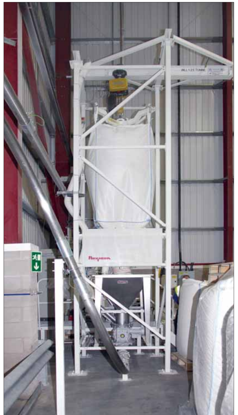
Pneumatic lines leading to and returning from tanker trucks make quick, clean work of discharging bulk bags for distribution of powdered ingredients
