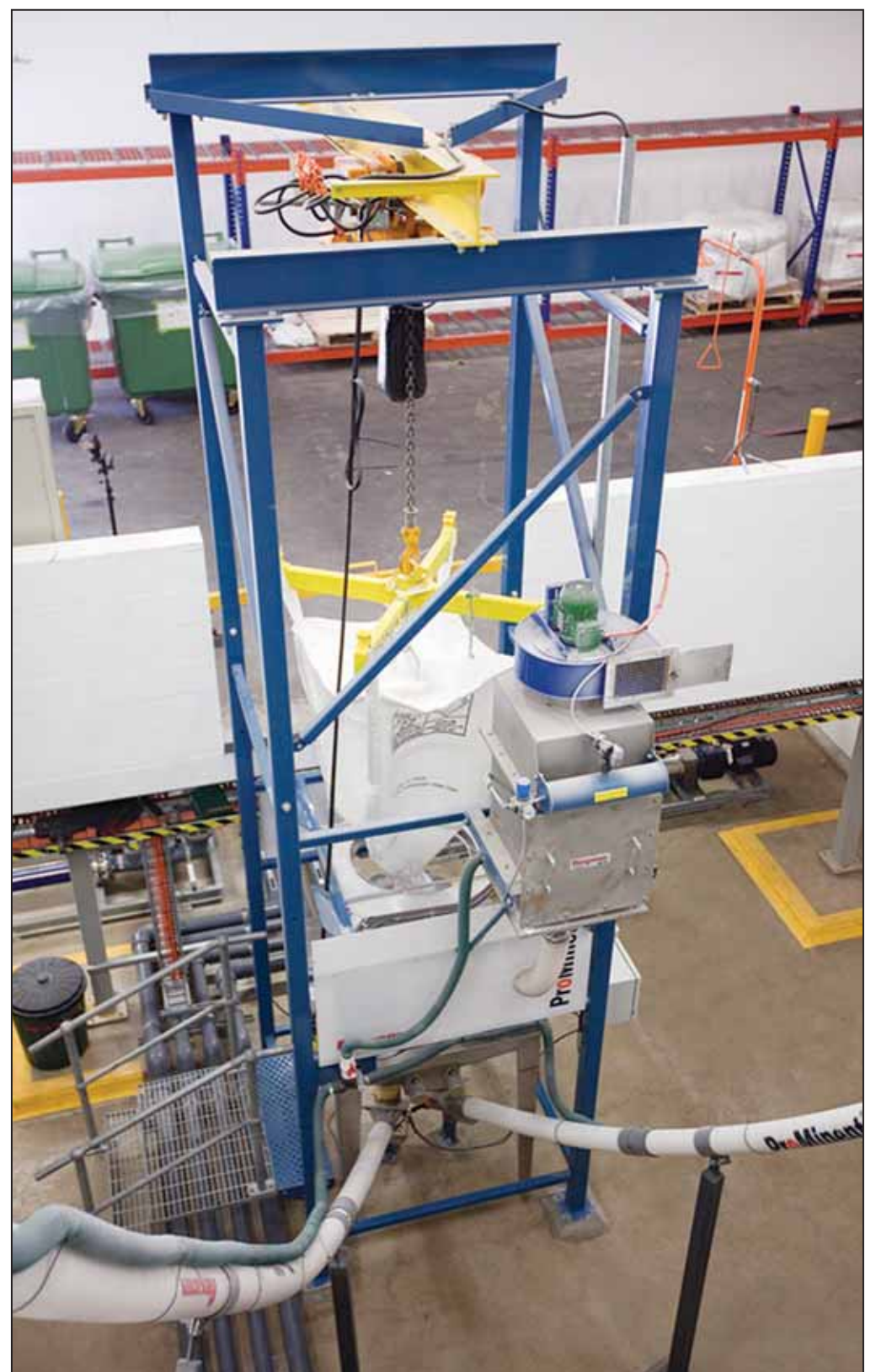
Powder remains enclosed from the time it is received until it enters the mixing tanks. The Bag-Vac dust collector, on the right of the discharger frame, prevents any dusting during bag loading, and removal and collapsing of empty bags
