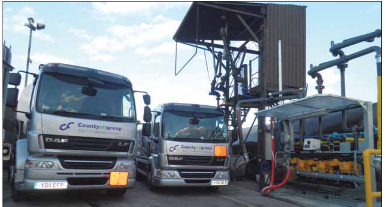
The new three-arm loading skid was configured for loading rated of 900 lpm
