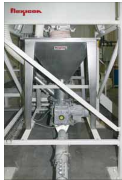
Raw material is gravity fed from the hopper through a rotary airlock with a pick-up adapter for discharge into a pneumatic line leading to a tanker truck loading bay
