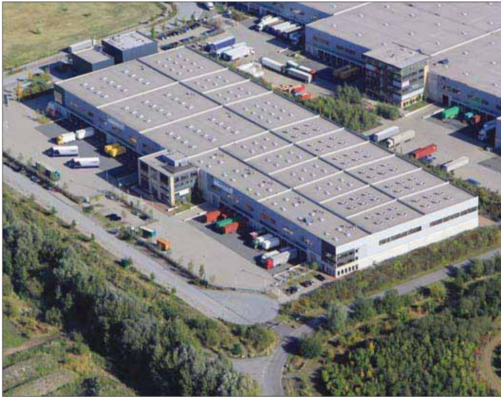
Lehnkering's has constructed a temperature-controlled storage unit at its dangerous goods warehouse at Hamburg-Altenwerder
