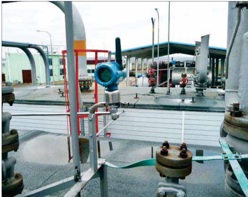
Wireless measurement devices have increased visibility into the process, enabling RWE to improve control and run closer to capacity
