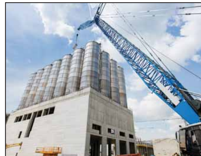
Talke successfully finished erecting 28 silos at the Slovnaft project
