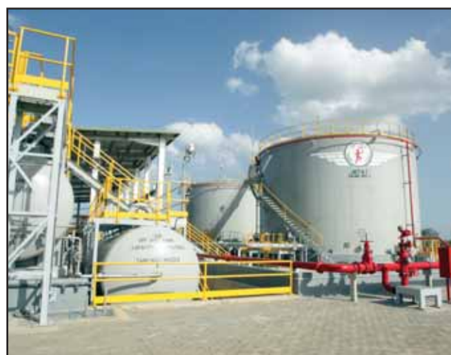
The Hambantota tank farm has a capacity of 80,000 cbm
