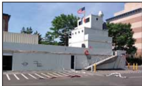
The New York Fire Dept. commissioned the construction of a shipboard firefighting simulator
