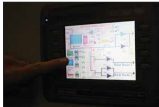
When Sven Beeusaert sets the chemical-dosing rate at the Cleaning Thys facility, a series of four aluminium Wilden Advanced Series A.025 AODD Pumps are called into action.
