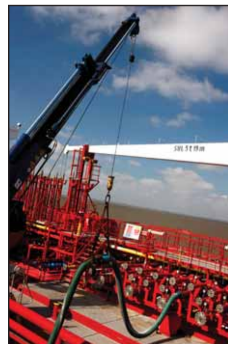
Harvest AVGAS 100LL is received by sea into the Immingham East Terminal via a dedicated flexible hose linked to a stainless steel import line
