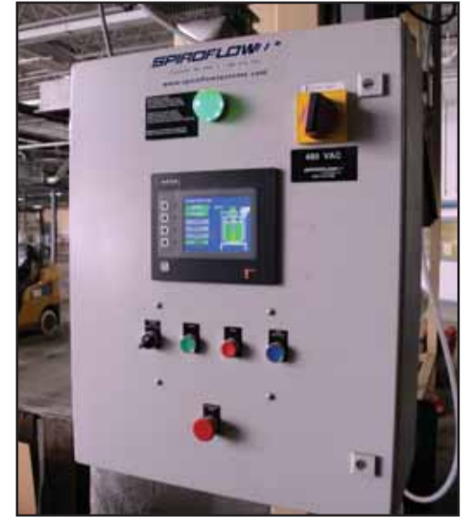
Spiroflow bulk bag filler gain-in-weight control panel
