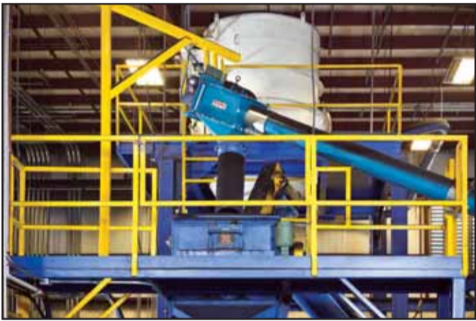
At the discharge end of the flexible screw conveyor, forward of the electric motor, ground particles gravity feed through a transition adapter and downspouting into the micro mill
