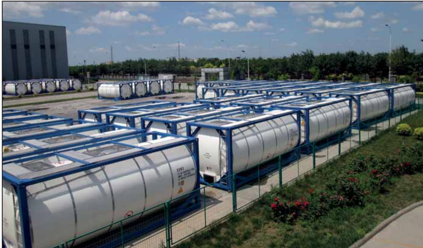
So far, data show that the chance of SCC on tank containers can be reduced by up to 10 times, MCC says
