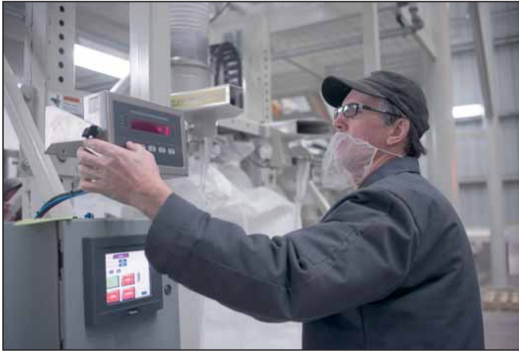
Once the operator connects the bag and pushes 'start' a PLC automates the filling process, closing the dome valve when the bag reaches its target weight
