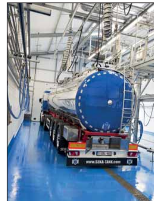
Tank truck in the wash bay
