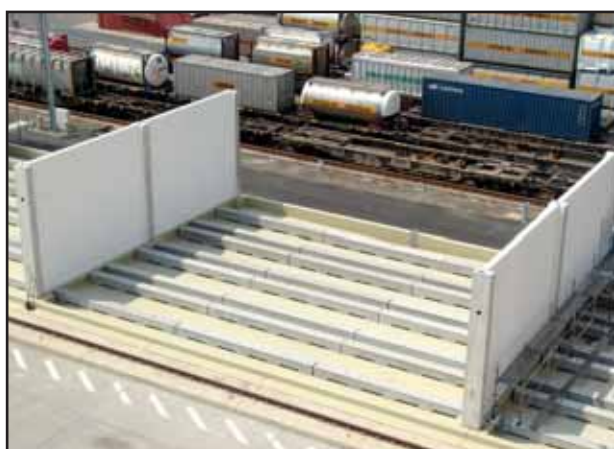
Mobile concrete walls allow the separation of hazardous goods categories
