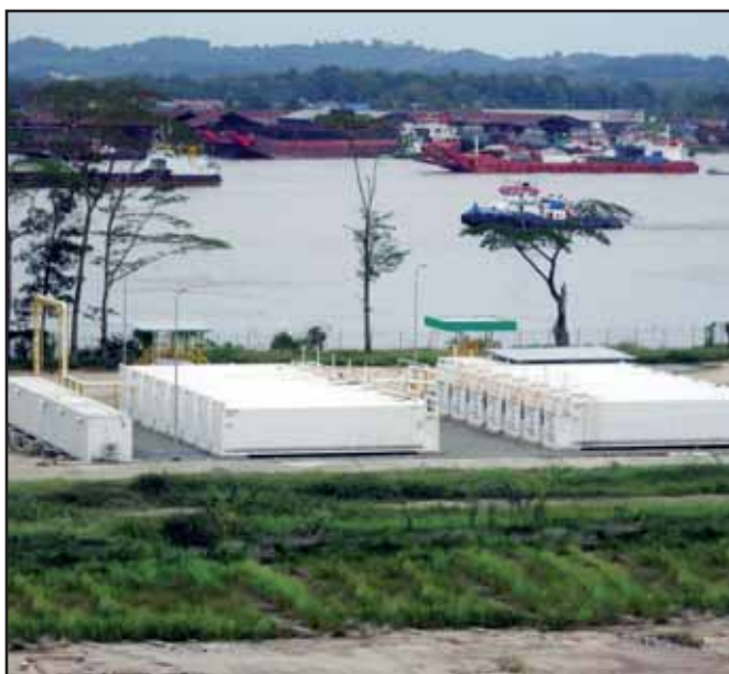
The portable tanks are simply moved into place and interconnecting pipework is installed
