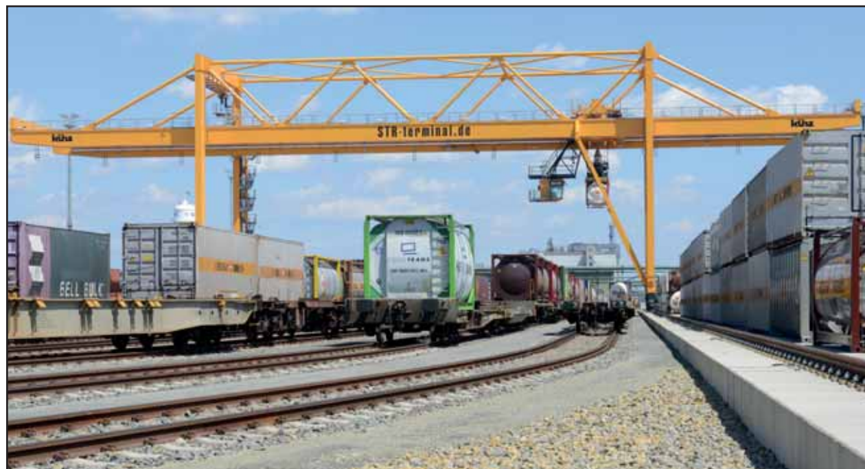
The STR expansion includes a second crane runway with six railway tracks
