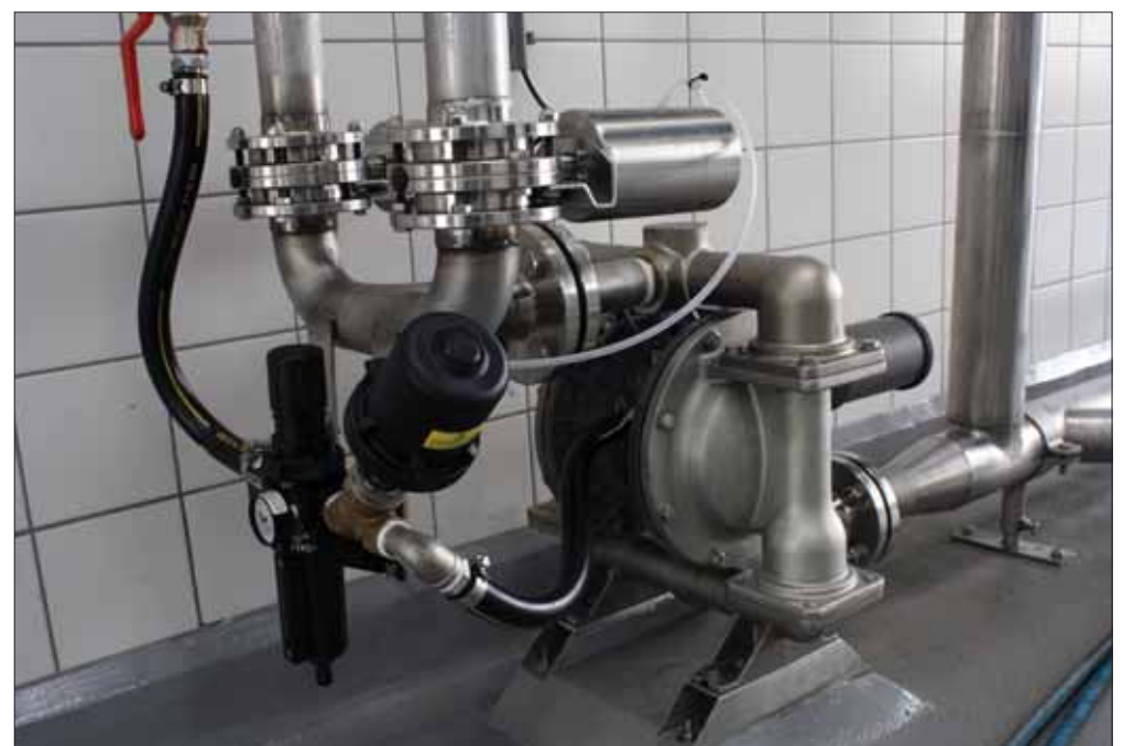
Chemical usage is one of the main cost considerations in tank cleaning and Wilden AODD pumps offer leak-free operation and accurate dosing that helps optimise that chemical usage
