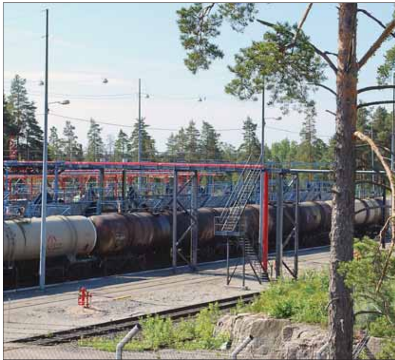
The rail yard at Neste Oil's refinery in Porvoo handles 20,000 tank wagons a year. It has the capacity to enlarge its operations, but Neste Jacobs' modelling tool clearly showed that not all crude is suited to rail transport. Pic © Neste Jacobs
