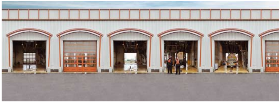
The new cleaning bays at Den Hartogh Botlek
