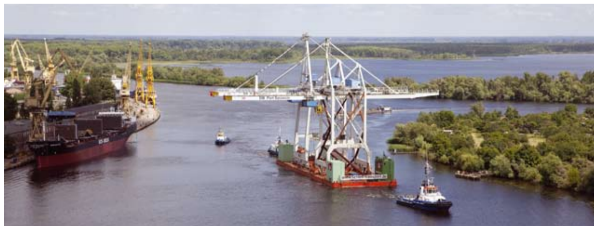
Two new gantry cranes have been installed in Szczecin. Pic DB Port Szczecin
