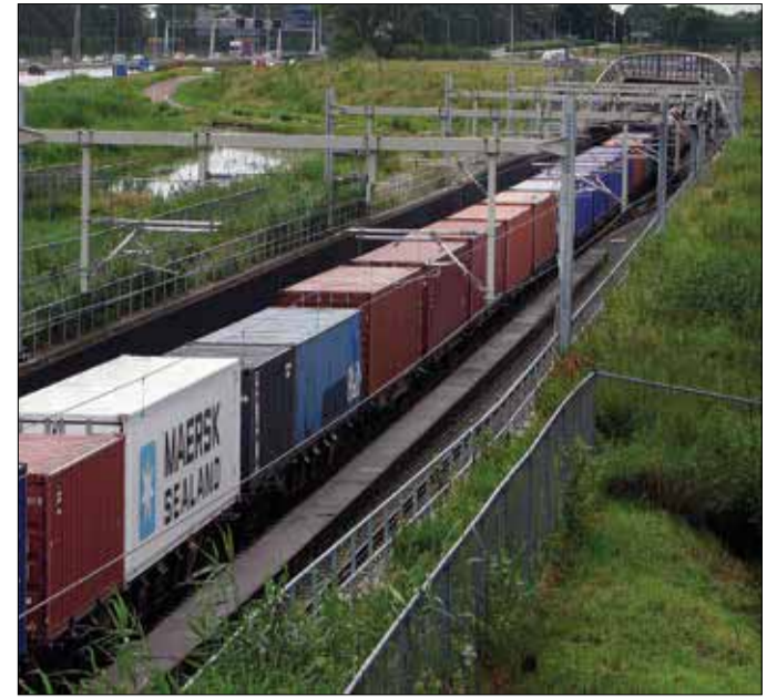
A third rail line between Emmerich and Oberhausen is an important milestone in the extension of the Betuweroute
