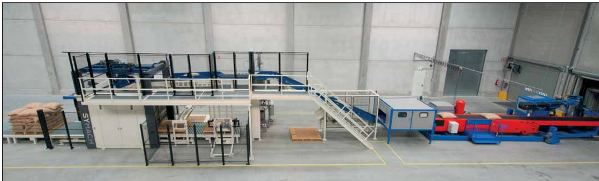
The Copal C2 bags handling line
