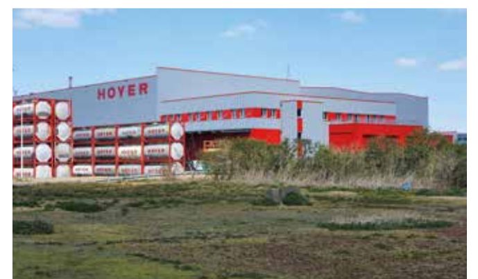
Hoyer's new logistics centre in the Dormagen Chempark
