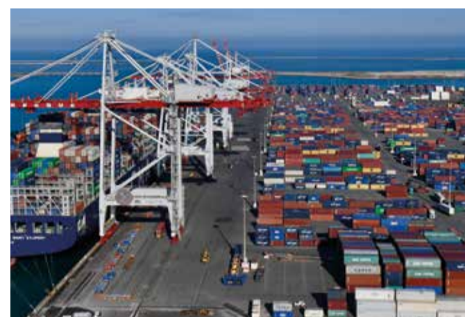
The year was marked by the commissioning of the extension to the quai de Flandre
