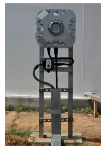
GroundGuardian detects hazardous changes in resistance of the electrical bond between the floating roof and the storage tank's grounding system
