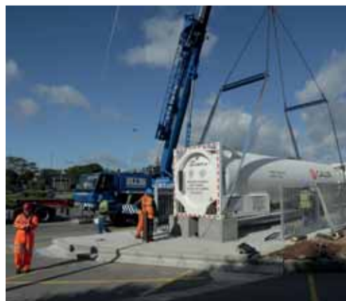
The new system uses 'zero loss' cooling technology to keep LNG within the storage tank at the ideal temperature and pressure which reduces the likelihood that warm gases such as methane need to be vented
