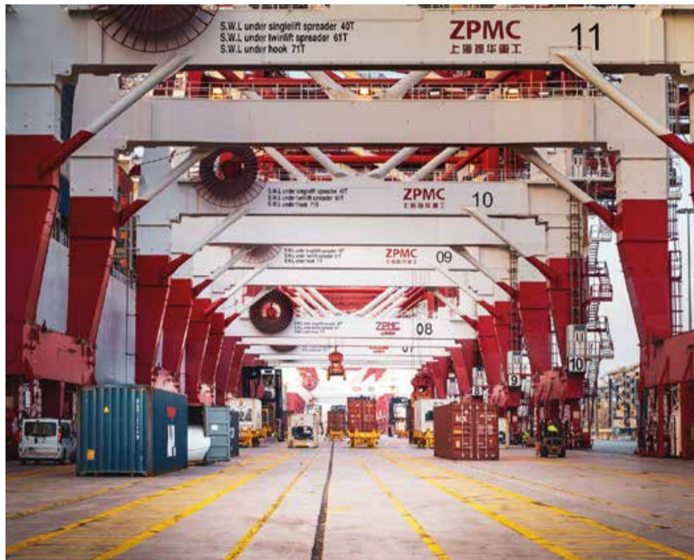
BEST's reefer related services will reduce in/out transport costs and related CO2 emissions, the terminal operator says
