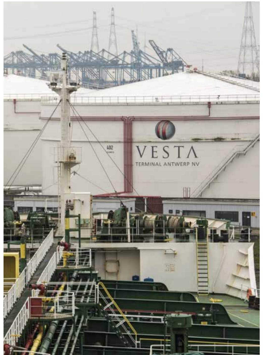
Vesta's expansion consists of five new tanks of 30,000 cbm each
