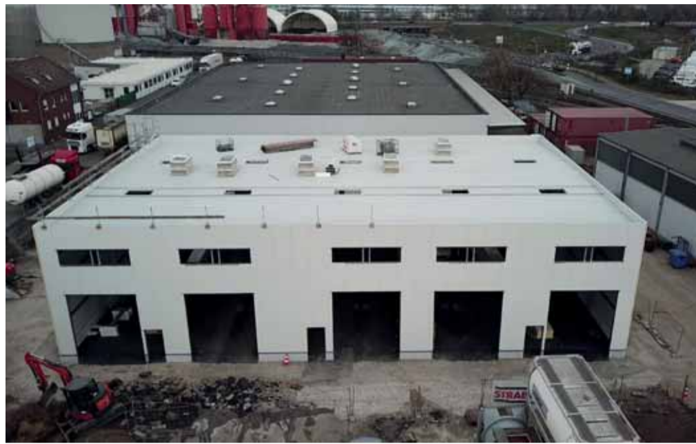
Filzhut's cleaning station in Neuss will be completed in August this year and will be equipped with a system from Gröninger Cleaning Systems
