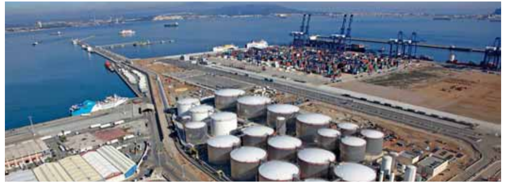
Vopak's Algeciras terminal is one of three European facilities the company is selling to First State
