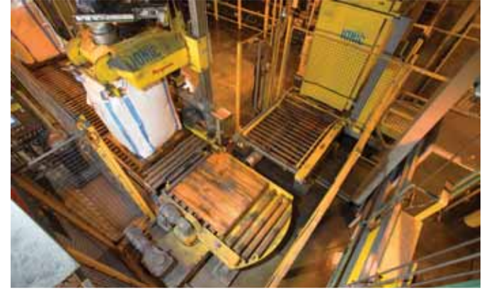
An automated pallet dispenser feeds pallets to the bulk bag filler which receives copper concentrate granules from the 11 ton capacity hopper above
