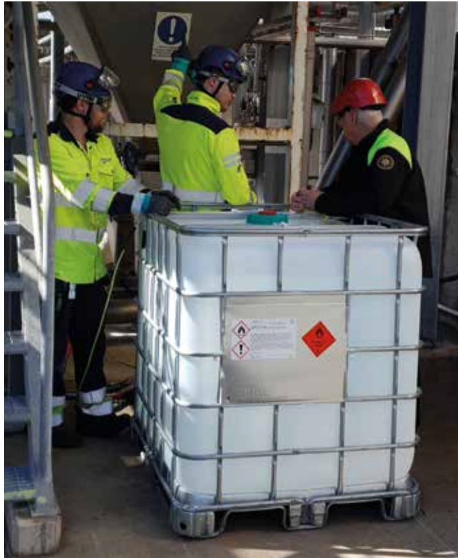
The metal cages containing the plastic IBC should be grounded (as it appears to be here)
