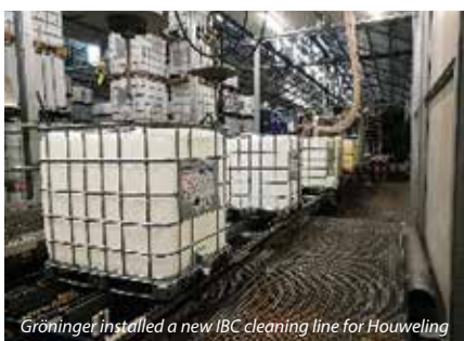
Gröninger installed a new IBC cleaning line for Houweling
