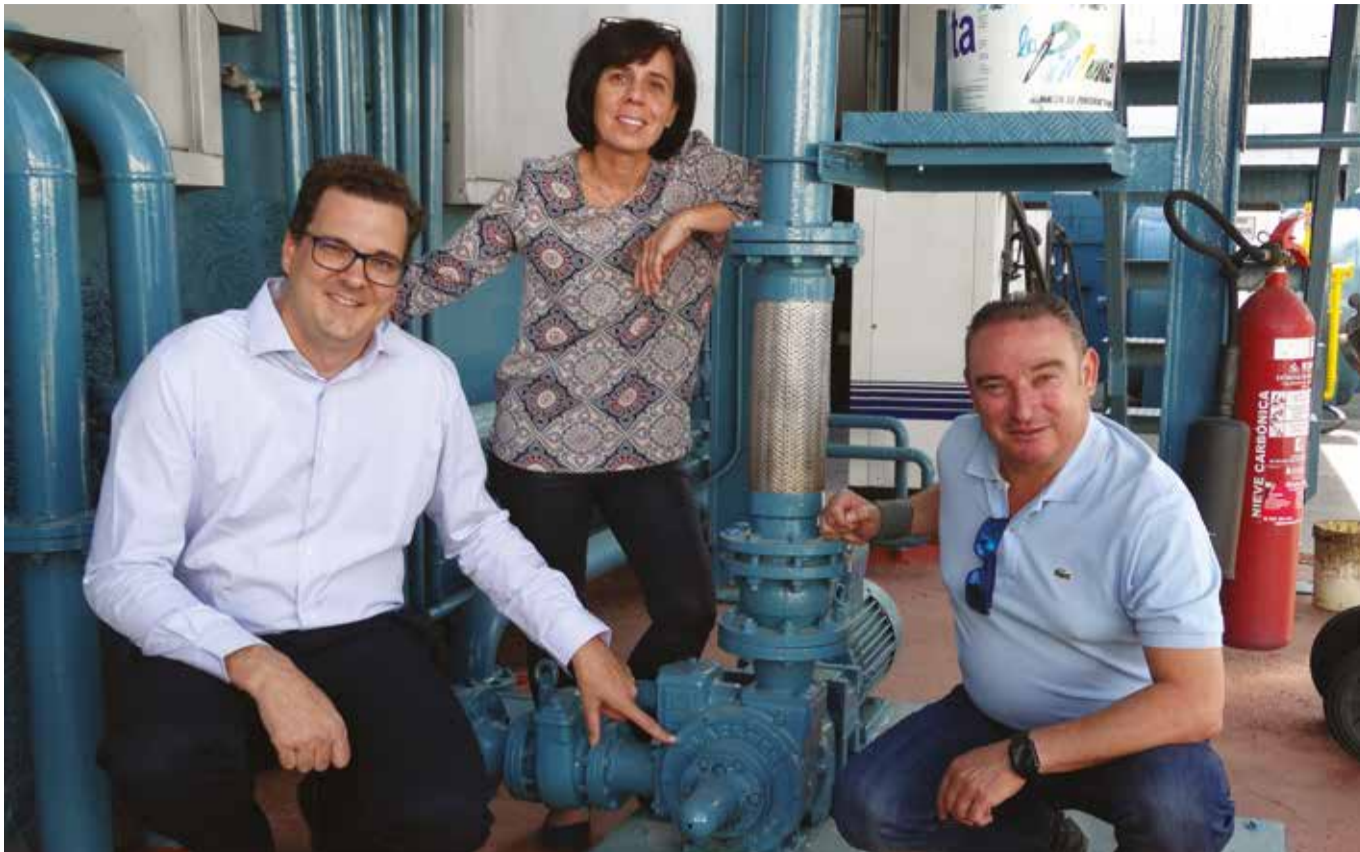
With the assistance of Marcos Kremers, left, sales manager of Cetil Dispensing Technology, and Iris Willmes, centre, regional sales manager for PSG and Blackmer, Ángel Reques, Jr, right, and his Reques e Hijos fuel distribution business has become the leading supplier of heating oil and diesel fuel in the Madrid market
