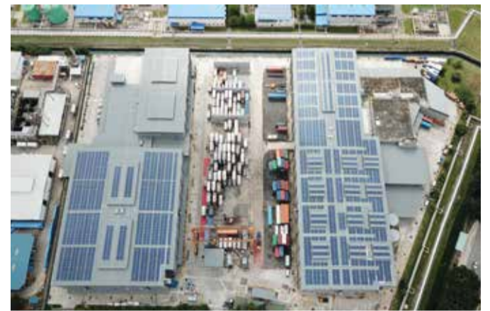
44,000 sqm photovoltaic system at Bertschi's chemical logistics centre in Singapore
