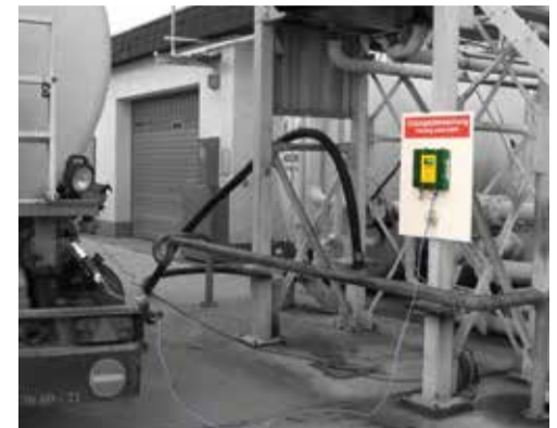
Fig 4. Grounding monitoring of a truck by means of Farado
