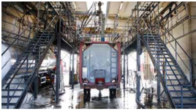
Last year, Van Moer invested over €2.8 million in the renovation of its cleaning tracks
