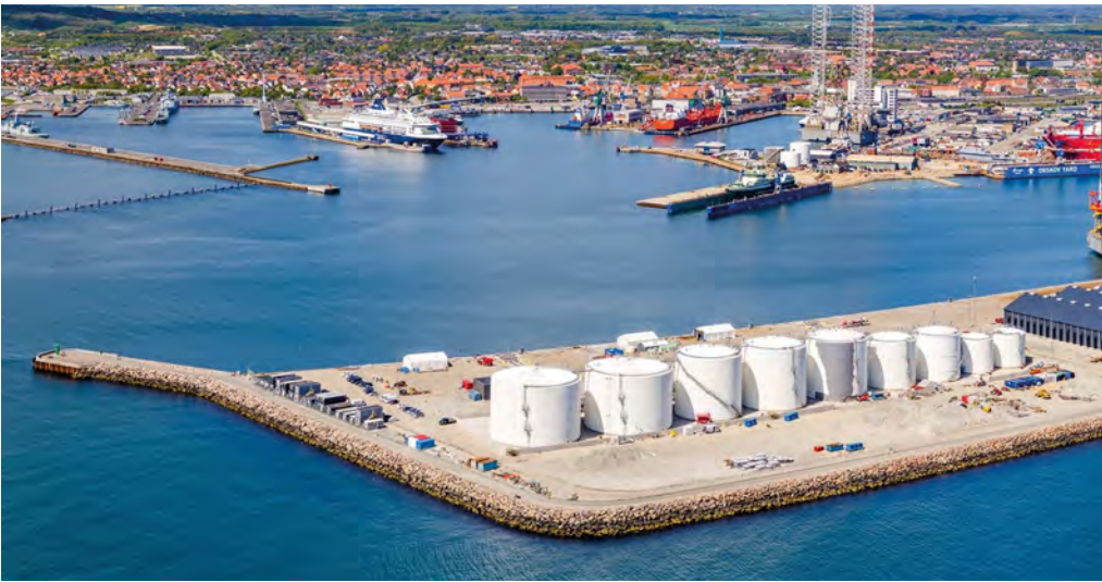
Stena’s Frederikshavn terminal has a capacity of 75,000 cbm
