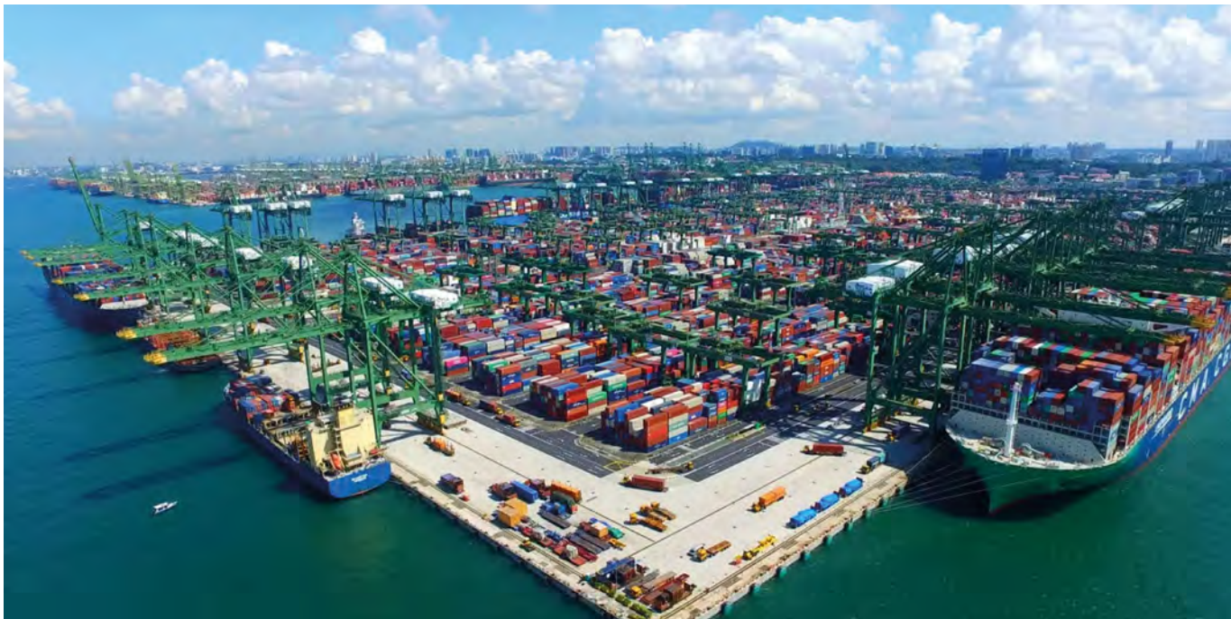
PSA operates the world's largest container transshipment hub
