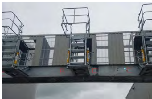
For another IFC customer, an existing platform for tanker loading was upgraded to include a fall prevention system
