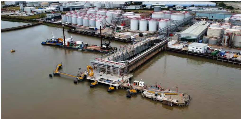
The new jetty has been constructed over the old structure, which was built in the 1900s
