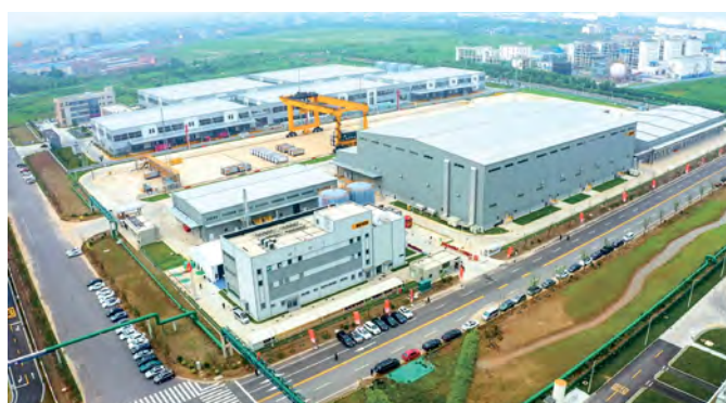
Last year, Bertschi opened its Zhangjiagang Liquids Chemical Hub
