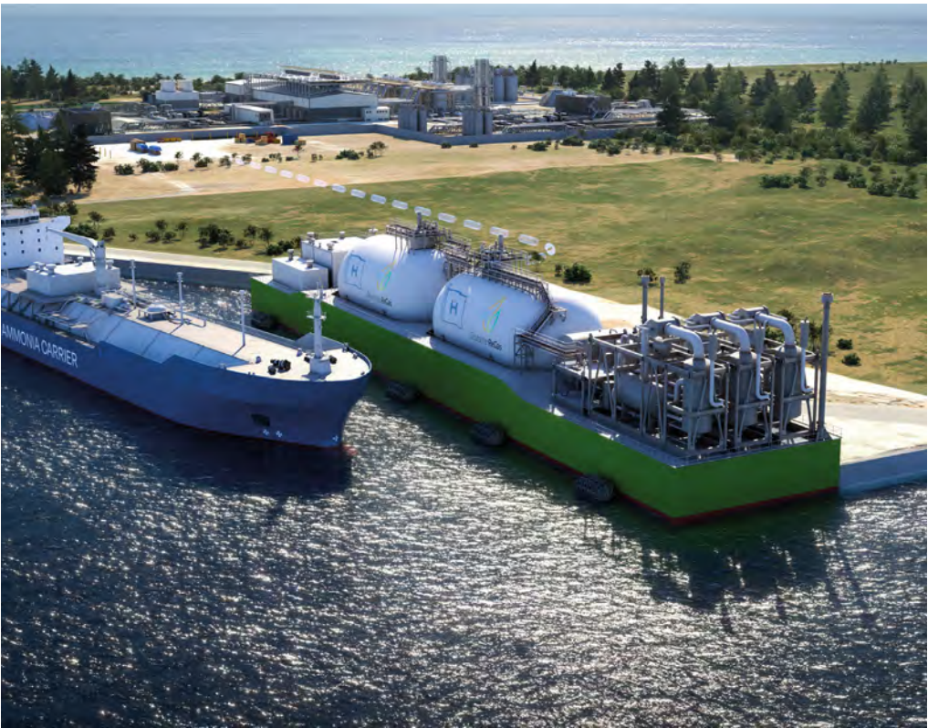
The terminal will be the world's first floating green ammonia cracker, producing around 30,000 tons of hydrogen a year
