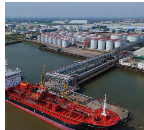
Stolthaven Terminals acquired the Dagenham facility in 2012 and it has since been extensively modernised and expanded
