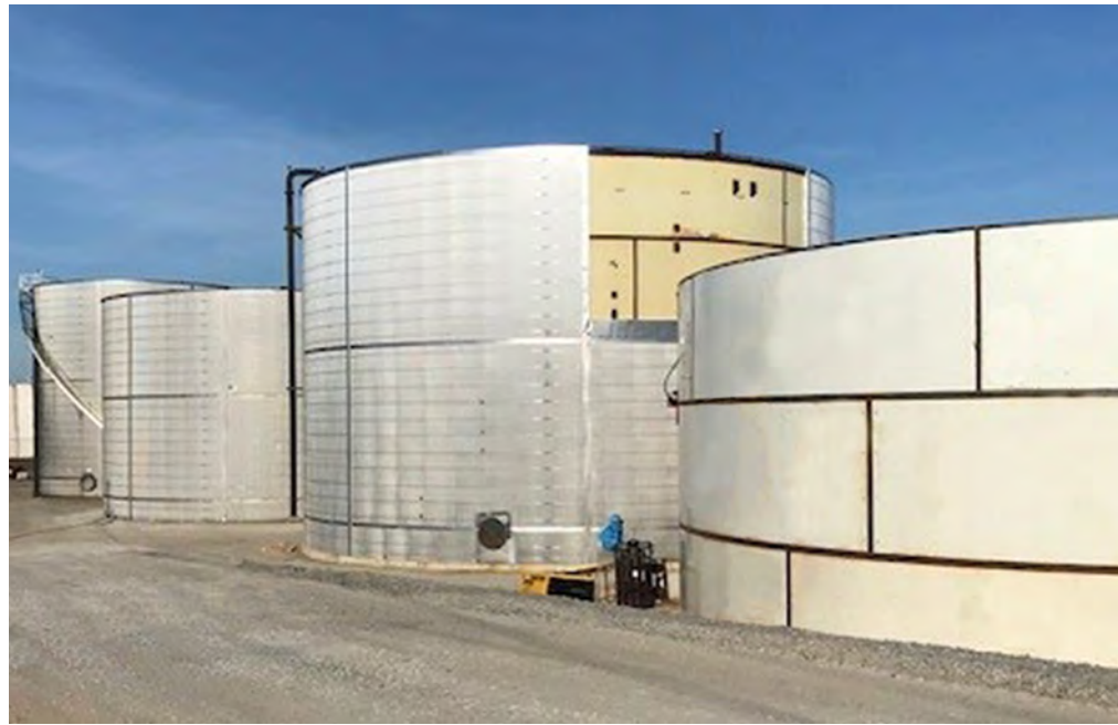
At Tanco Burns Harbor, the contrast between a completed steel tank without insulating wrap (right) and wrapping nearly complete (left)
