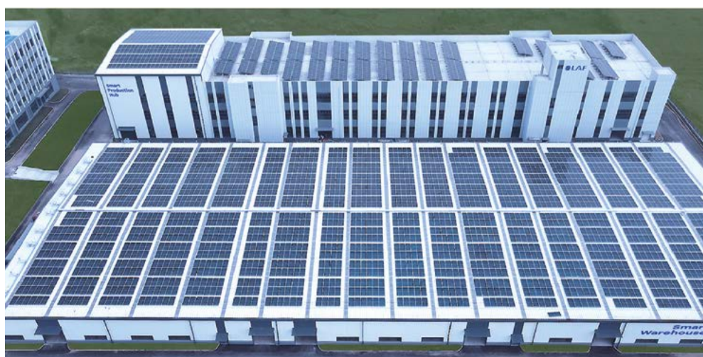
Monocrystalline solar photovoltaic system
