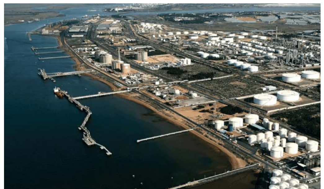
The Exolum infrastructure will serve a new biofuels plant at the La Rábida Energy Park
