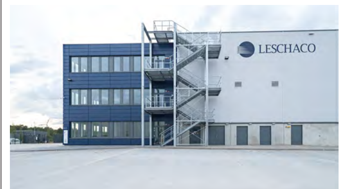
A key differentiator of the site is its dedicated hazardous goods infrastructure
